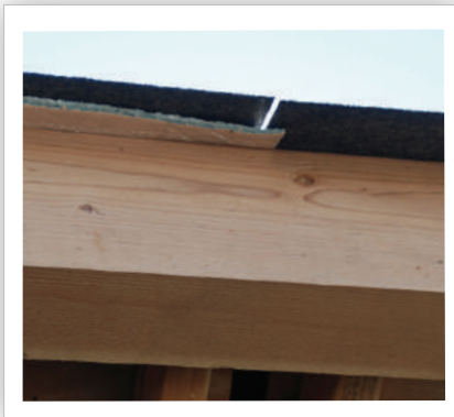
Therma Sheet under asphalt shingles
