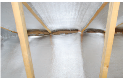
Attic Floor & Tab Insulation
